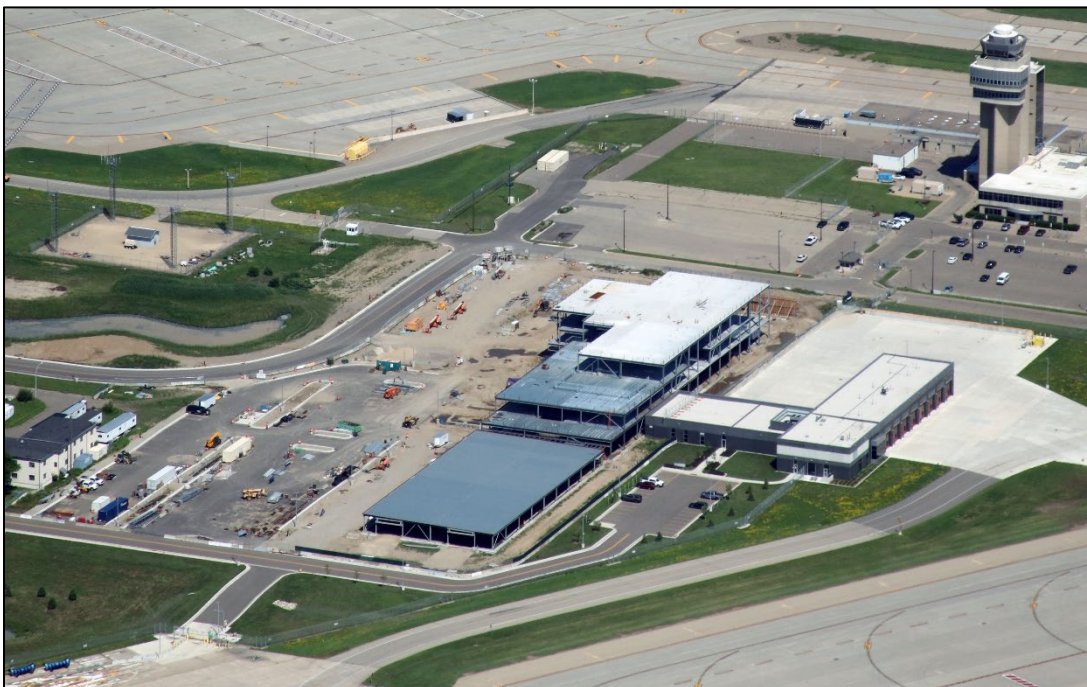
MSP Safety and Security Center Construction
