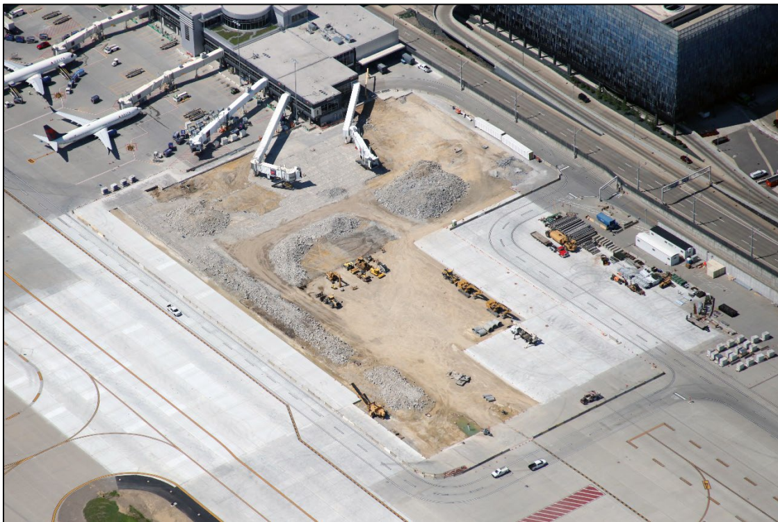
MSP Concourse G Apron and Taxiway B
