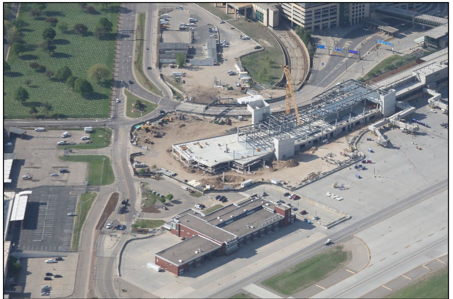
MSP Terminal 2 North Gate Expansion
