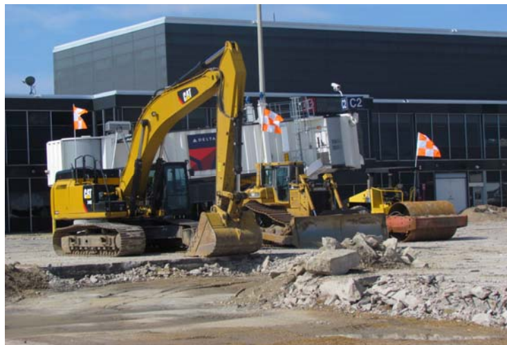
Pavement Repair outside C Concourse of Terminal 1-Lindbergh
