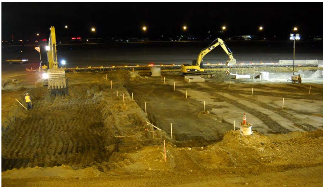
Terminal 1 C Concourse Apron Pavement Replacement
