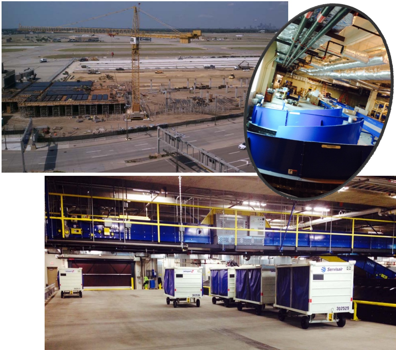
The New Baggage Handling/Inspection Building at Terminal 2-Humphrey
