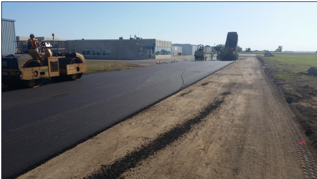
Flying Cloud Airport Taxiway Reconstruction
