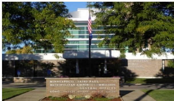
Metropolitan Airports Commission General Office
