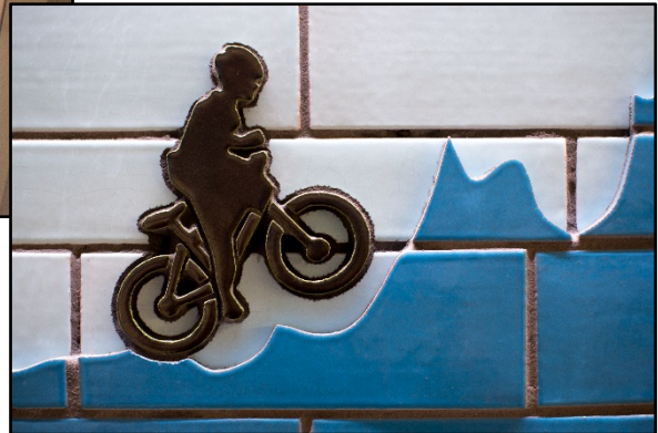
Detail of Custom Mosaic in Remodeled Restroom
