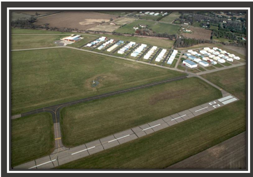
Lake Elmo Airport Taxiway Reconstruction
