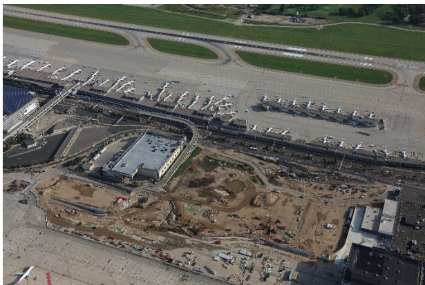
Terminal 1-Lindbergh Roadway Project
