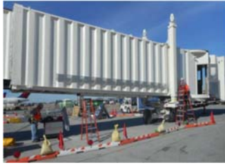
Passenger Boarding Bridge
