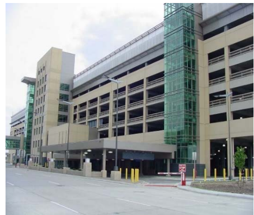
Parking Facility at MSP Terminal 2-Humphrey
