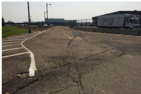
Landside Pavement to be Rehabilitated
