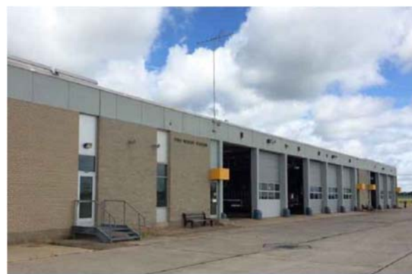
Aircraft Rescue & Fire Fighting Station #2
