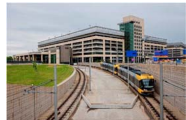
Terminal 2 Parking Ramp
