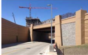
MAC Tunnel at MSP
