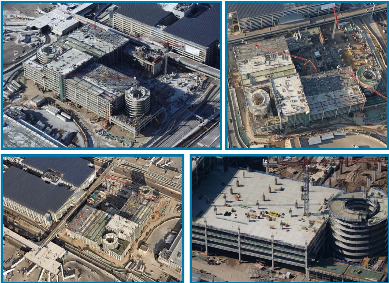
Progress Continues on the Silver Parking Ramp at Terminal 1-Lindbergh
