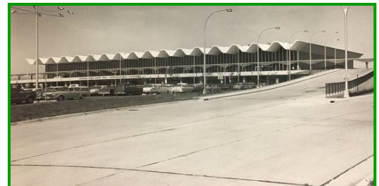
The New Terminal, Including Its Iconic Sawtooth Roof, Opens at MSP in 1962
