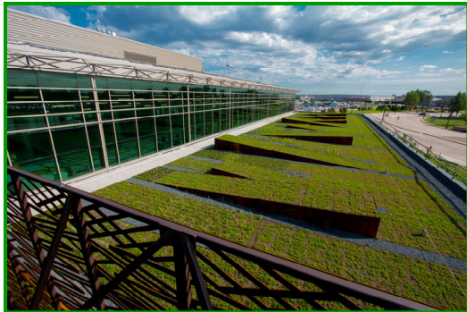
The 2016 Terminal 2 Expansion Includes Four New Gates, a Lactation Room, an Indoor Pet-Relief Area and a Green Roof
