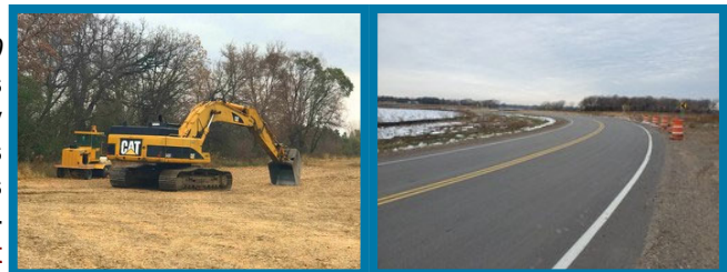
Lake Elmo Construction Replaces Runway 14-32, Adds Taxiways and Realigns 30 th Street
