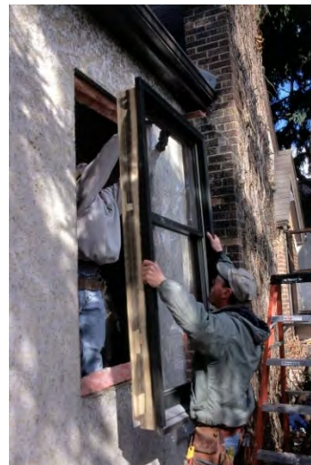
Window Replacement is One Component of Noise Mitigation
