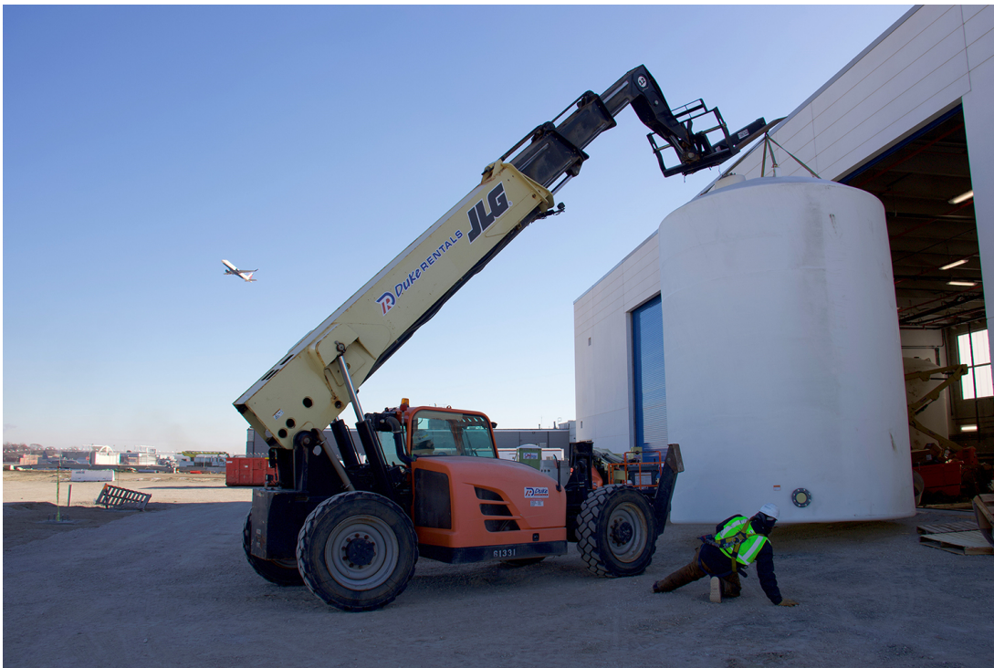
Field Maintenance Workers Installing New Deicer Tanks
