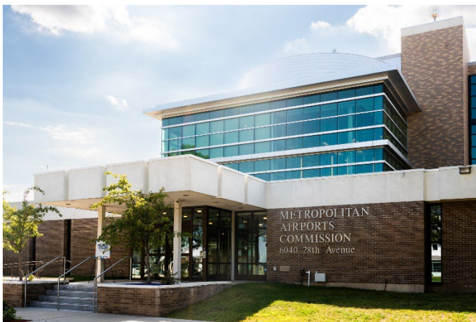
MAC General Office Building
