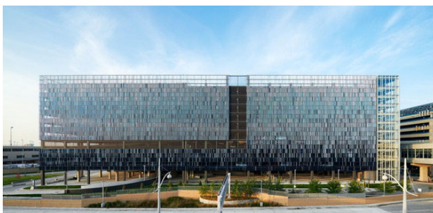
Bonds Provided Funds to Build the New Silver Ramp with its Beautiful Glazed Terracotta Baguette Exterior
