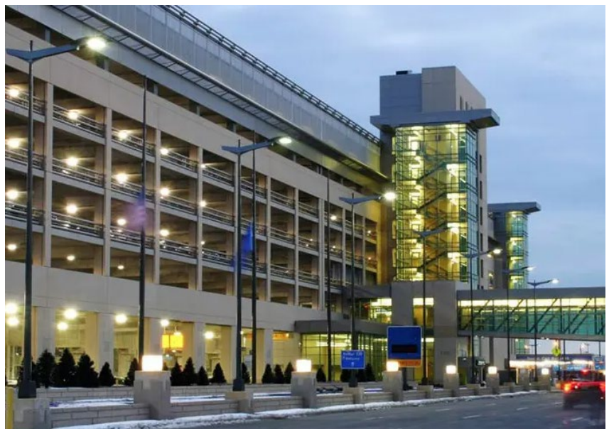
Building and Updating Parking Ramps at the MSP Airports are Typically Funded with Bond Proceeds
