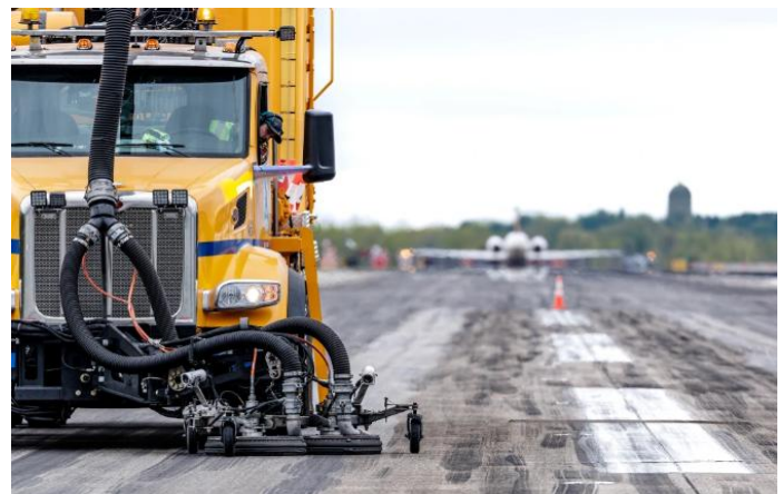
MSP Runway Construction
