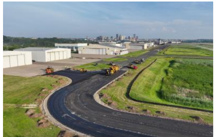
St. Paul Downtown Airport Runway Reconstruction in 2025
