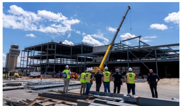
Constructing the Safety and Security Center
