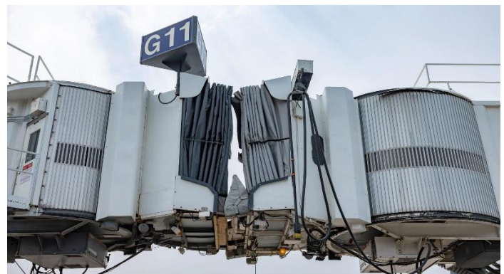
Boarding Bridges were Linked to Create a Temporary Secure Corridor for Passengers to Access MSP’s International Arrivals Facilities
