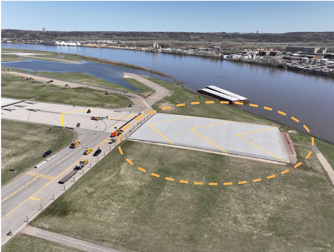
Image showing an example of EMAS at St. Paul Downtown Airport (STP)
