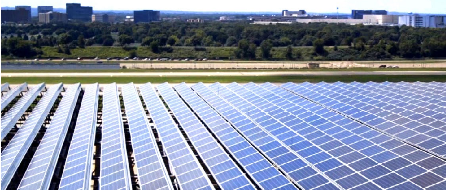
Solar Energy installation at Terminal 1-Lindbergh's parking facility.
