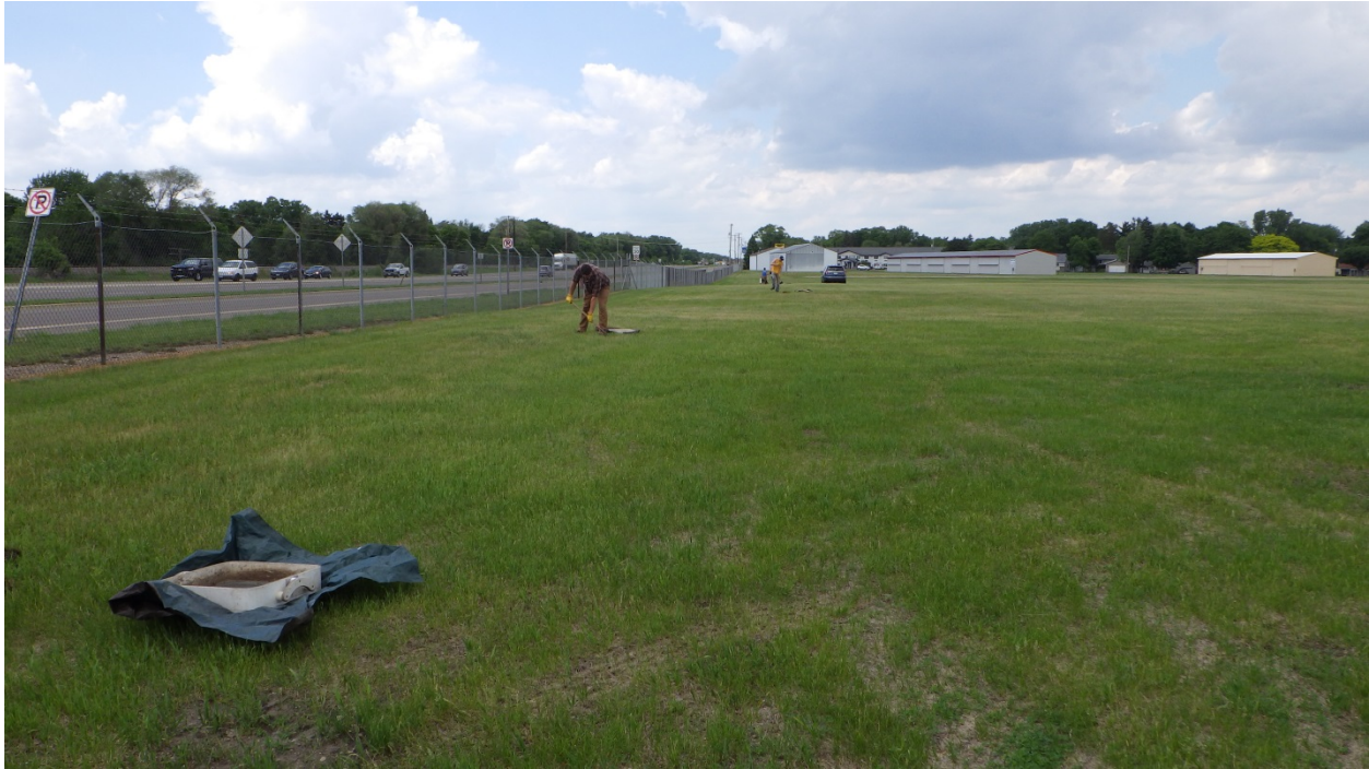
Figure 25. View from the southeast of survey in the footprints for the northwest corner of the apron expansion and the west perimeter road to its north.
