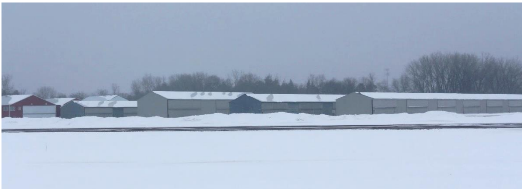
Figure 24. Overview of the west side of Hangar Area 3, view facing northwest.
