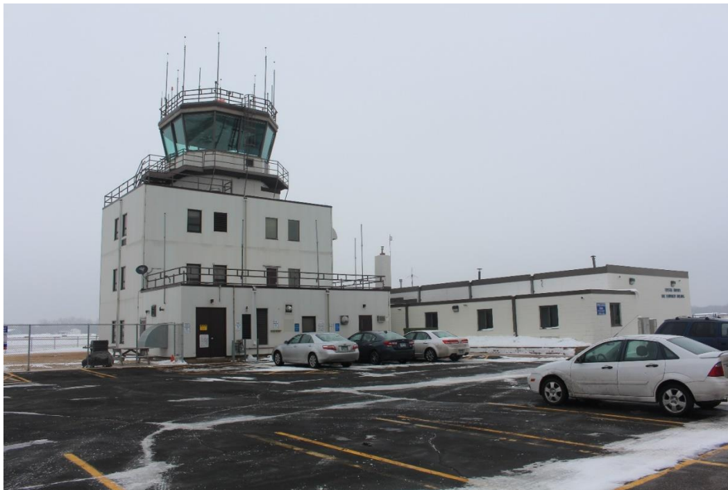
Figure 8. Crystal Airport terminal building and control tower, view facing northeast.
