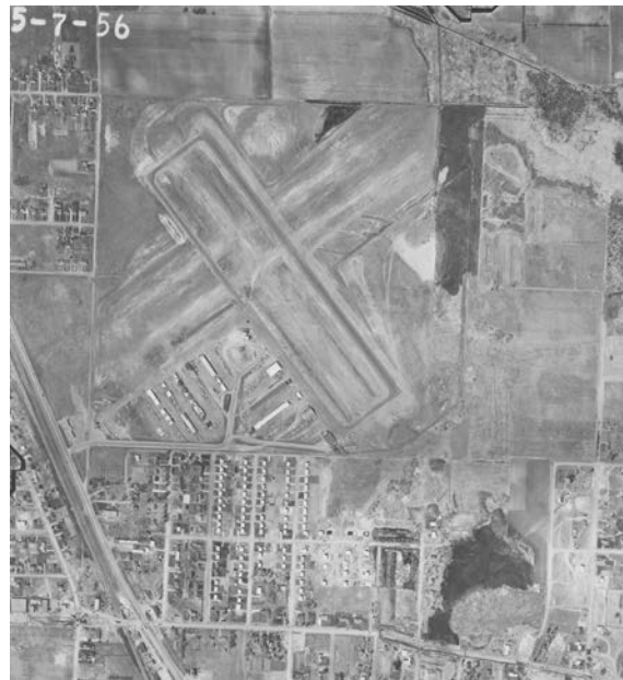
Figure 8. 1956 aerial photo showing early runways in a formation similar to the present. (University of Minnesota – Minnesota Historical Aerial Photographs Online HHJ-241).
