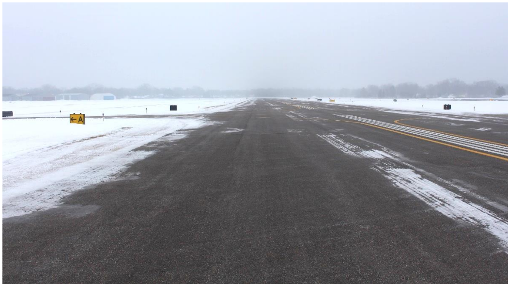
Figure 2. Paved Runway 14L/32R, view facing northwest.
