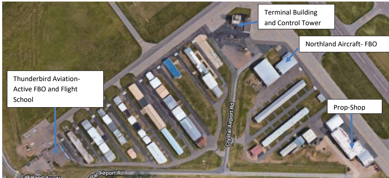
Figure 6. Current aerial of Hangar Area 1.
