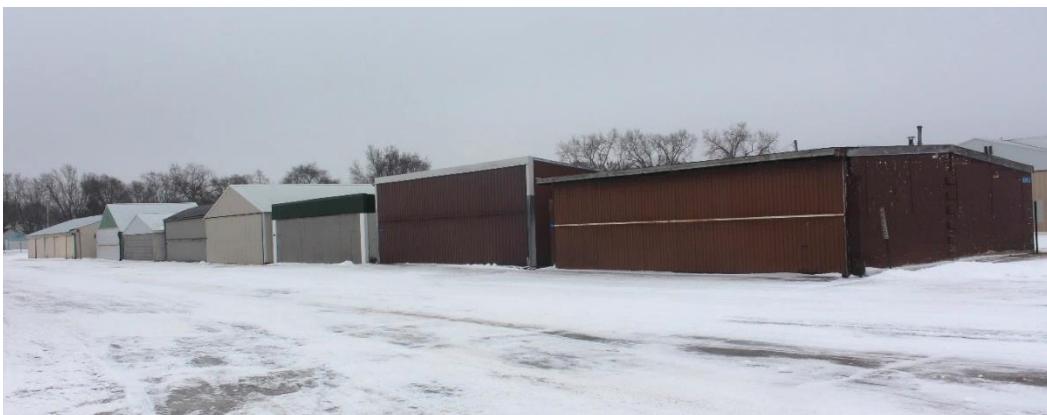
Figure 17. Row of 1950s and 1960s hangars on the west side of Hangar Area 1, view facing southwest.
