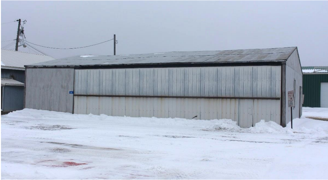
Figure 22. Ca. 1960 hangar in Hangar Area 2, view facing north.
