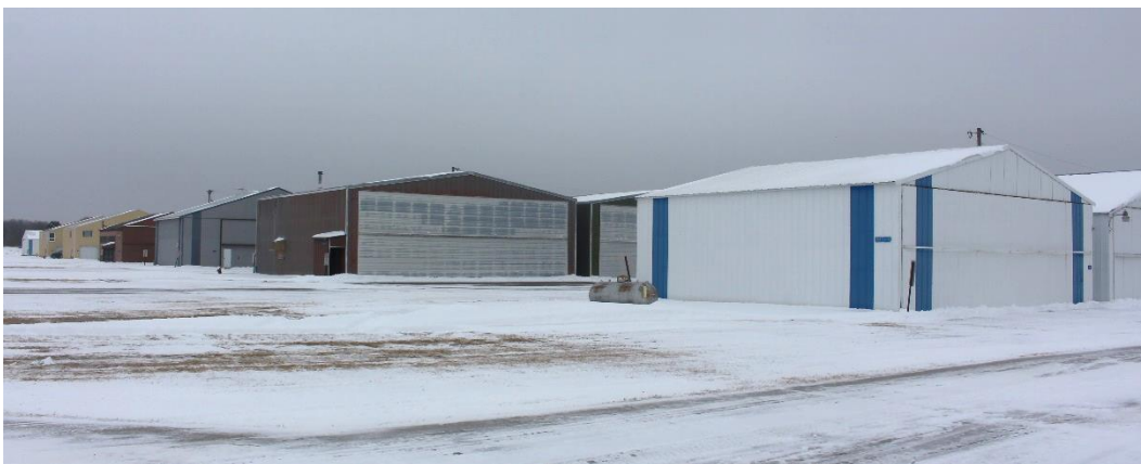
Figure 28. Hangar Area 4, view facing northeast.
