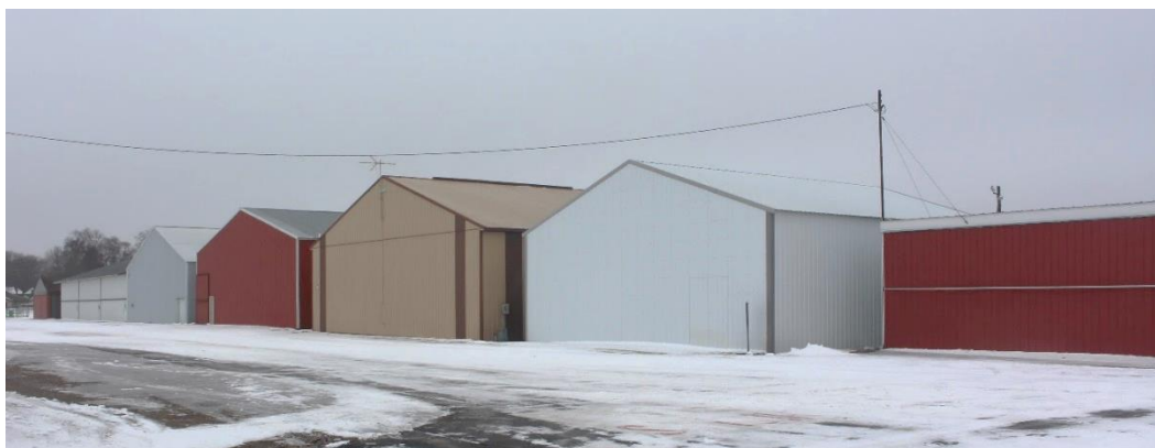
Figure 20. Ca. 1991 hangars on the west side of Hangar Area 1, view facing southwest.
