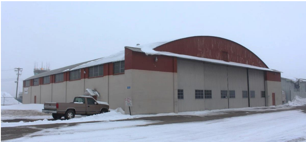
Figure 12. 1967 hangar associated with Northland Aircraft, view facing north.
