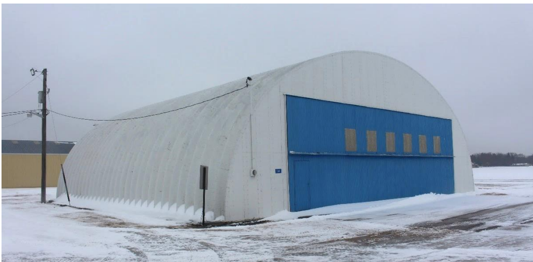
Figure 31. Ca. 1971 Quonset-style hangar, view facing southeast.
