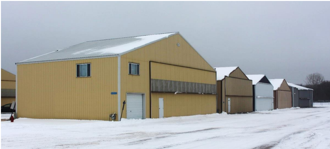
Figure 29. Row of 1990s hangars in Hangar Area 4, view facing northeast.
