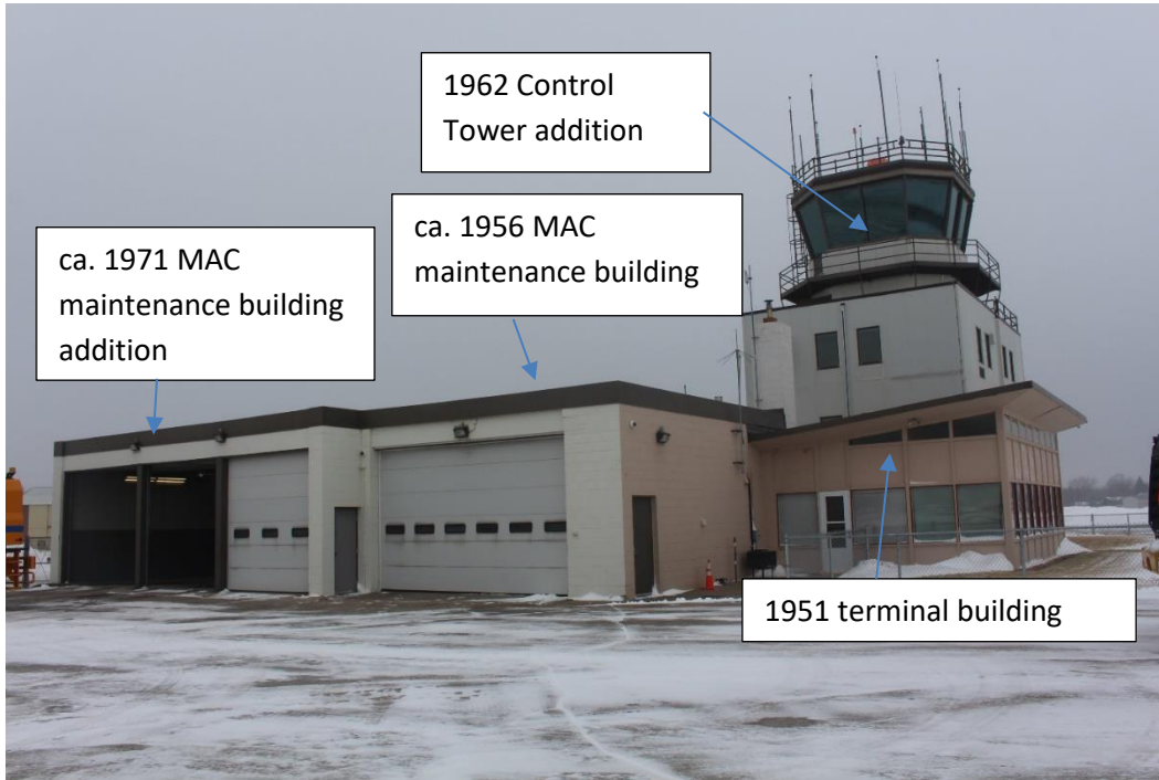
Figure 7. Crystal Airport terminal building and control tower, view facing southwest, showing the four components of the building: the 1951 terminal building, ca. 1956 MAC maintenance building, 1962 control tower, and ca. 1971 MAC maintenance building addition.
