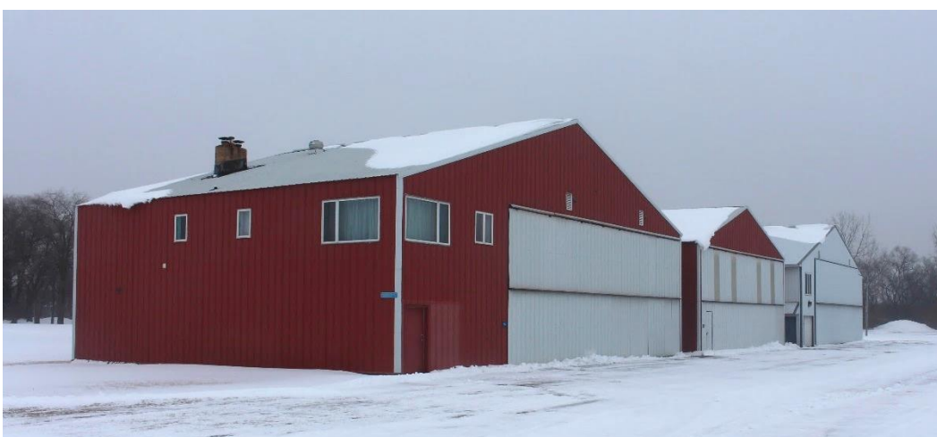
Figure 26. 1990s hangars in Hangar Area 3, view facing north.
