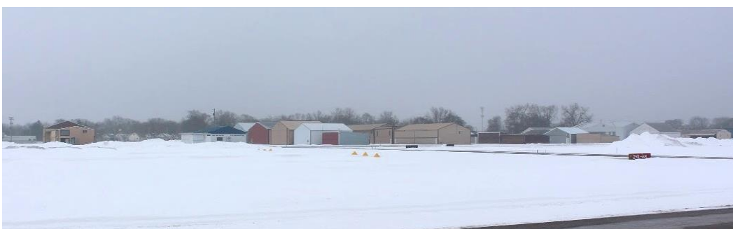
Figure 16. Overview of the west side of Hangar Area 1, view facing south.
