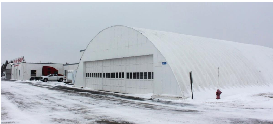
Figure 14. Prop-Shop, view facing southeast.
