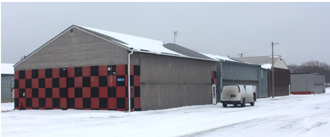
Figure 30. 1960s and 1970s hangars in Hangar Area 4, view facing northeast.
