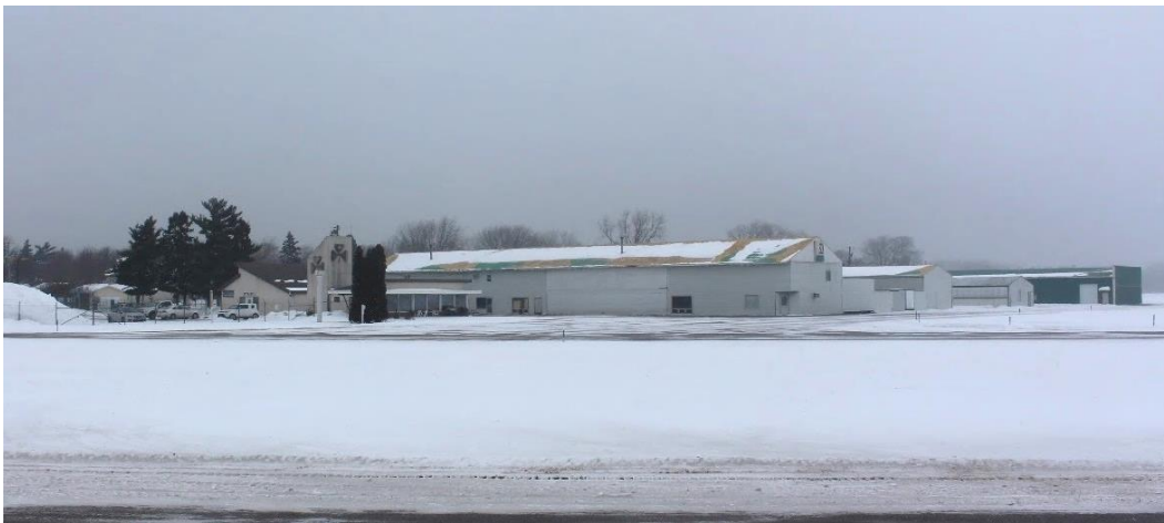
Figure 21. Overview of east side of Hangar Area 2, view facing north northeast.
