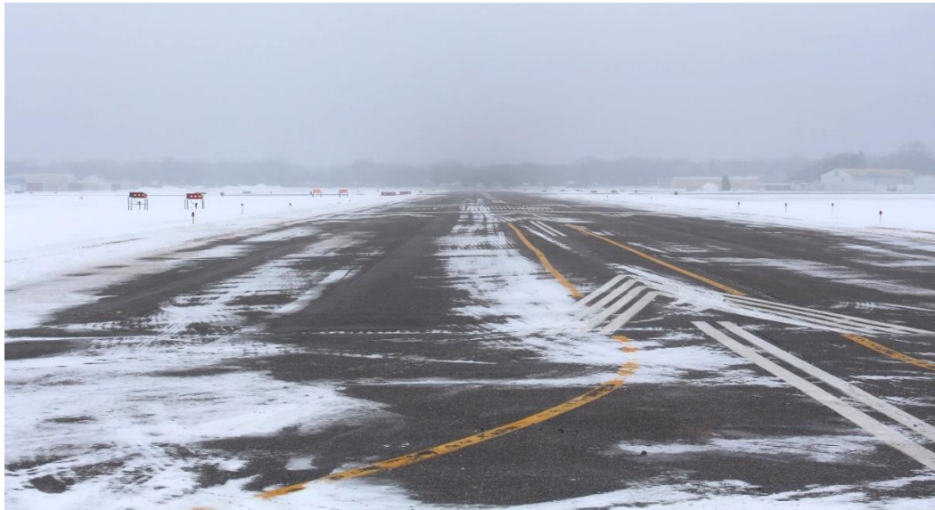
Figure 3. Paved Runway 6L-24R, view facing southwest.
