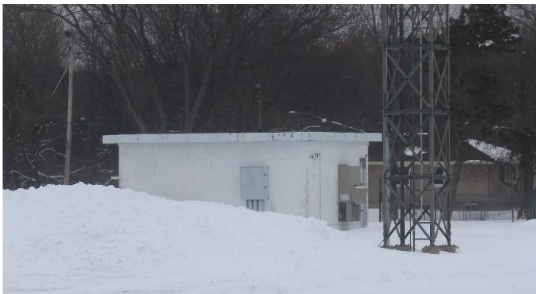
Figure 32. Ca. 1966 FAA radio equipment building, view facing east northeast.
