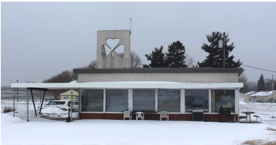
Figure 23. Ground service facility (former Crystal Shamrock FBO, ca. 1966), view facing west.
