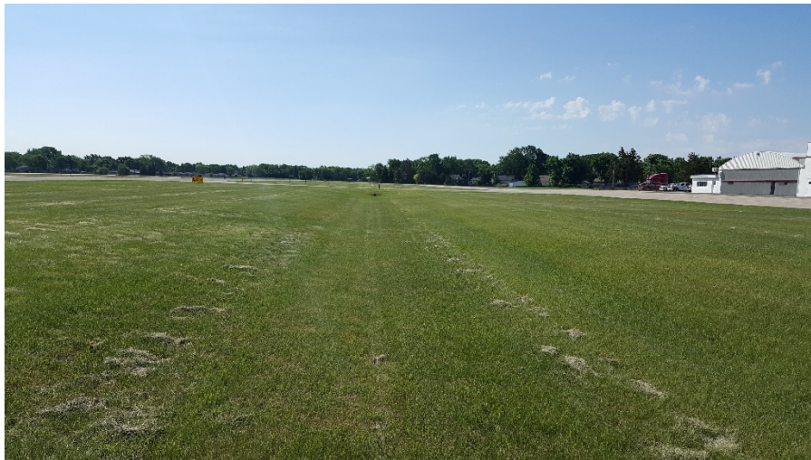
Photo 7. Taxiway connector. General infield, view to the southeast.
