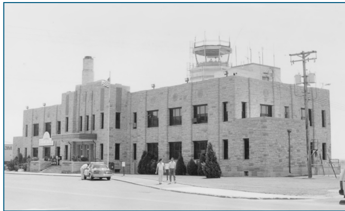
Historic STP Terminal Building
