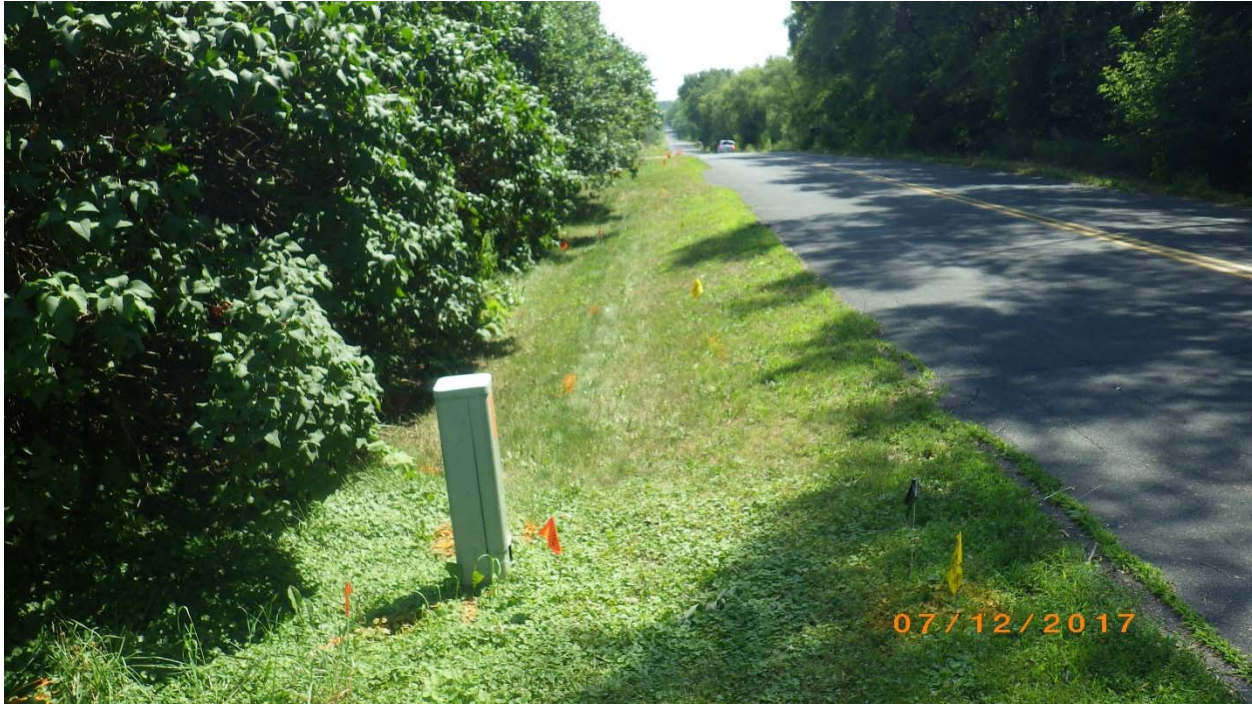
Figure 8. Example of utility disturbance east of Neal Avenue North. View facing south.
