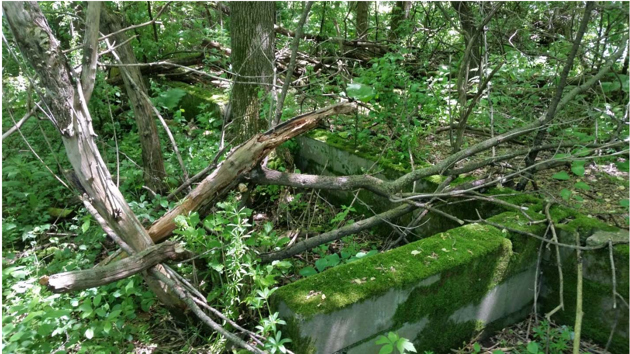
Figure 16. View of cinderblock foundation at 21WA0119.
