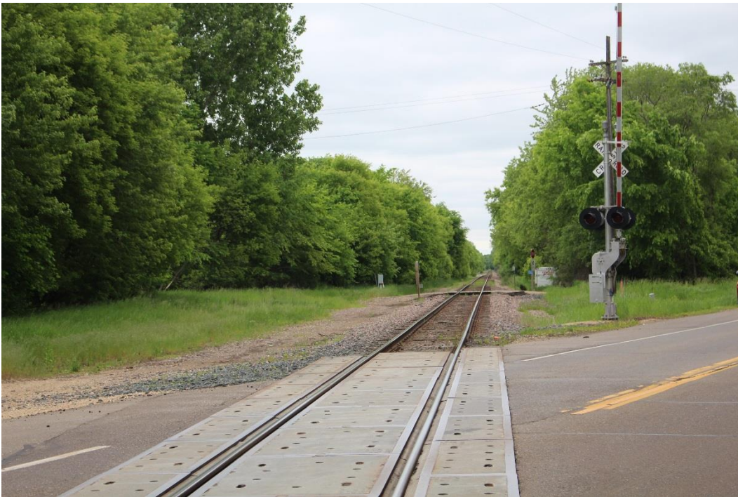
St. Paul, Stillwater & Taylor's Falls Railroad at intersection with 40 th Street N.
