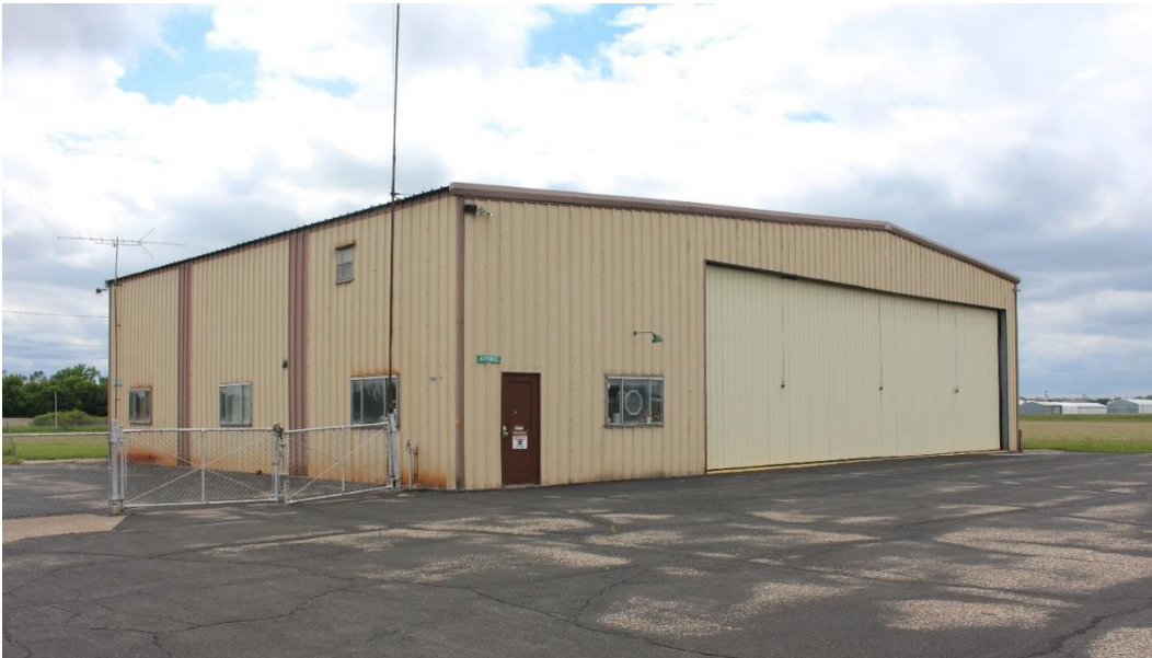
Figure 6. c.1970 south maintenance building, view facing southwest.
