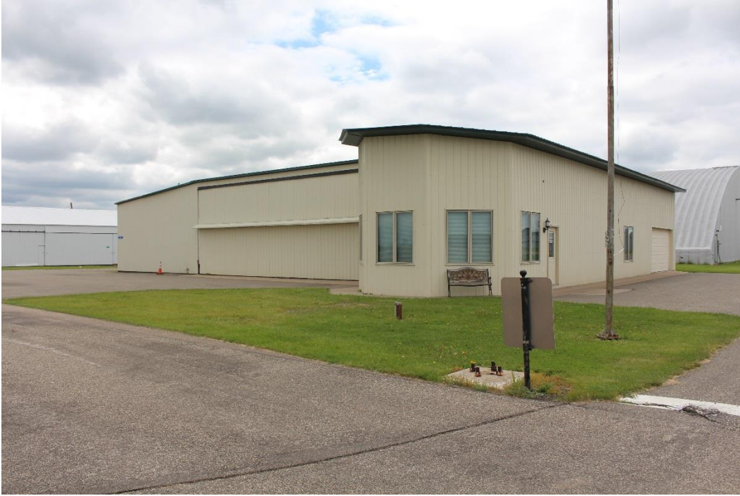
Figure 5. c.1960 building, possibly a former FBO building, view facing west.
