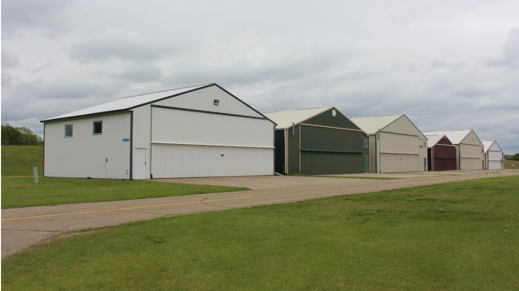
Figure 11. Modern box hangars, view facing southeast.
