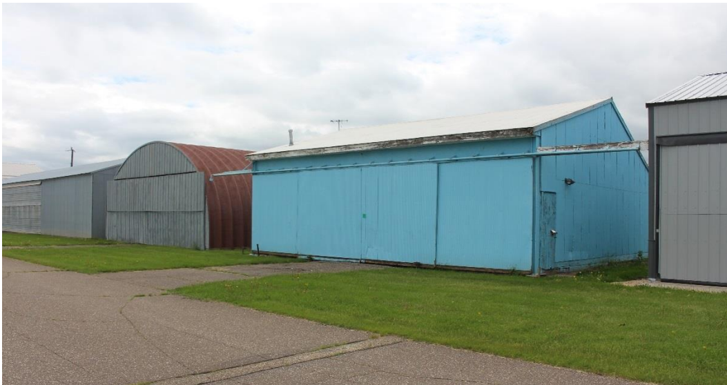
Figure 8. Historic-age Box and Quonset hangars, view facing south.
