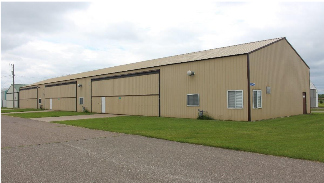
Figure 12. Modern box hangar, view facing southwest.
