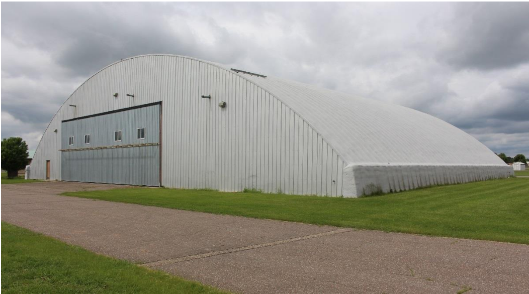
Figure 10. Large c.1970 Quonset Hangar, view facing north.
