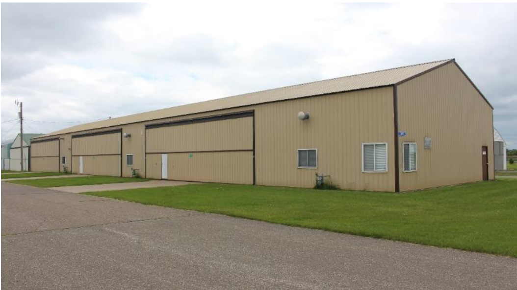
Modern box hangar, view facing southwest.
