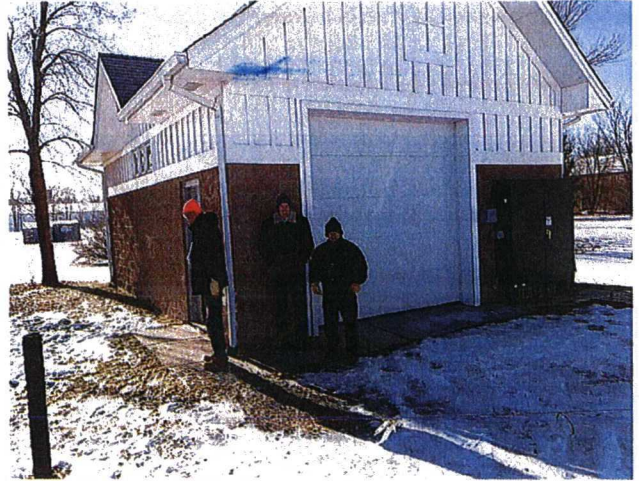
Building housing the source area air stripper (used to treat extracted source area groundwater; currently inactive to improve in-situ treatment effectiveness)
