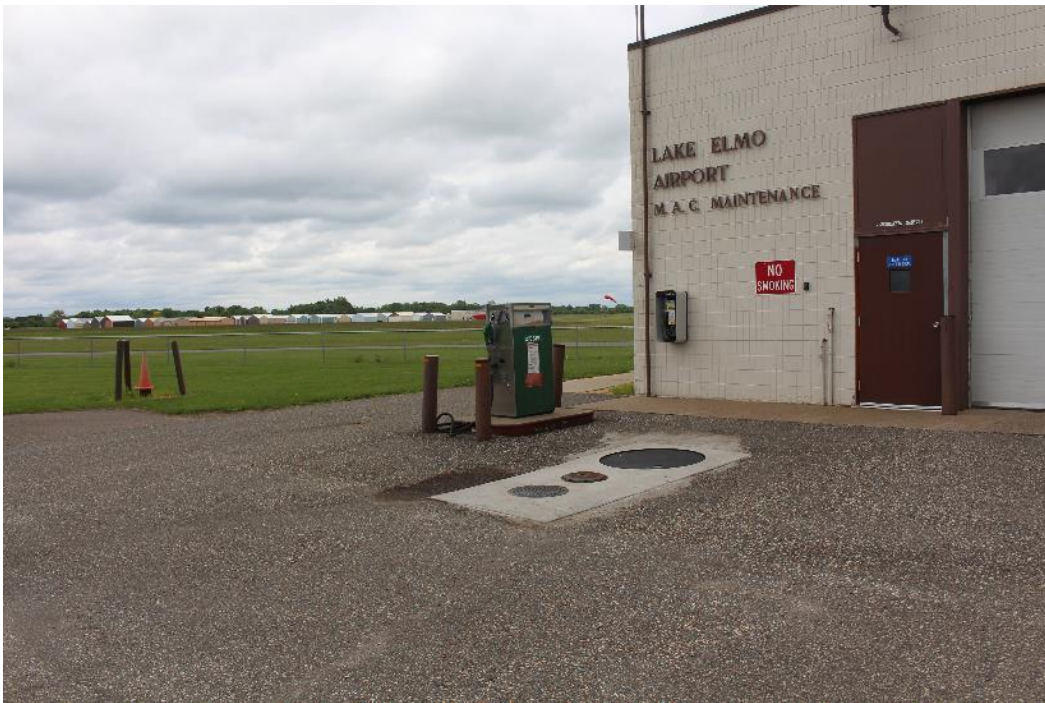
Diesel fuel pump and UST at MAC Maintenance Building.
