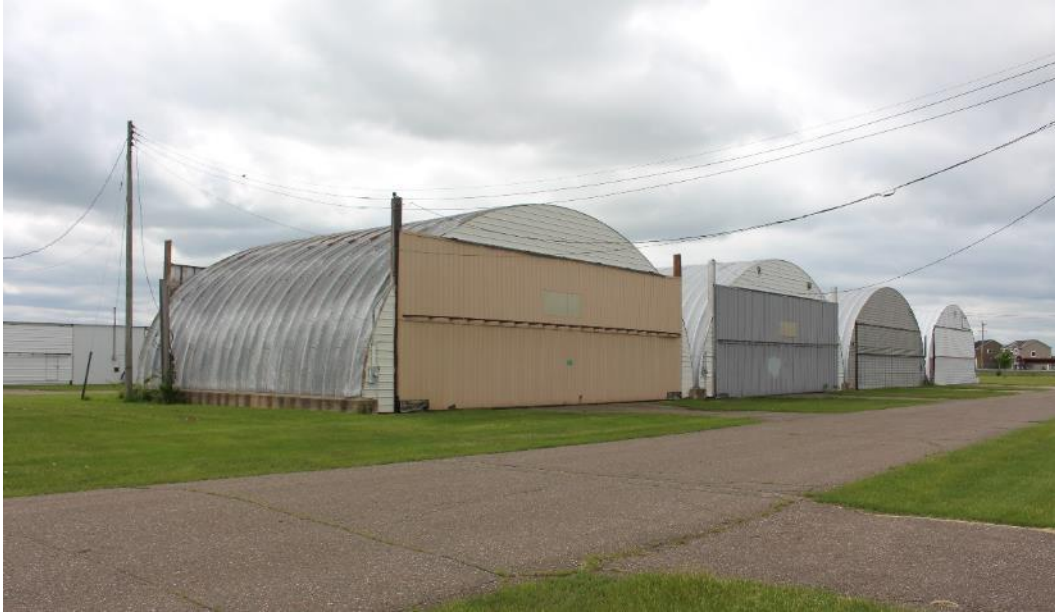
Historic-age Quonset hangars, view facing southwest.
