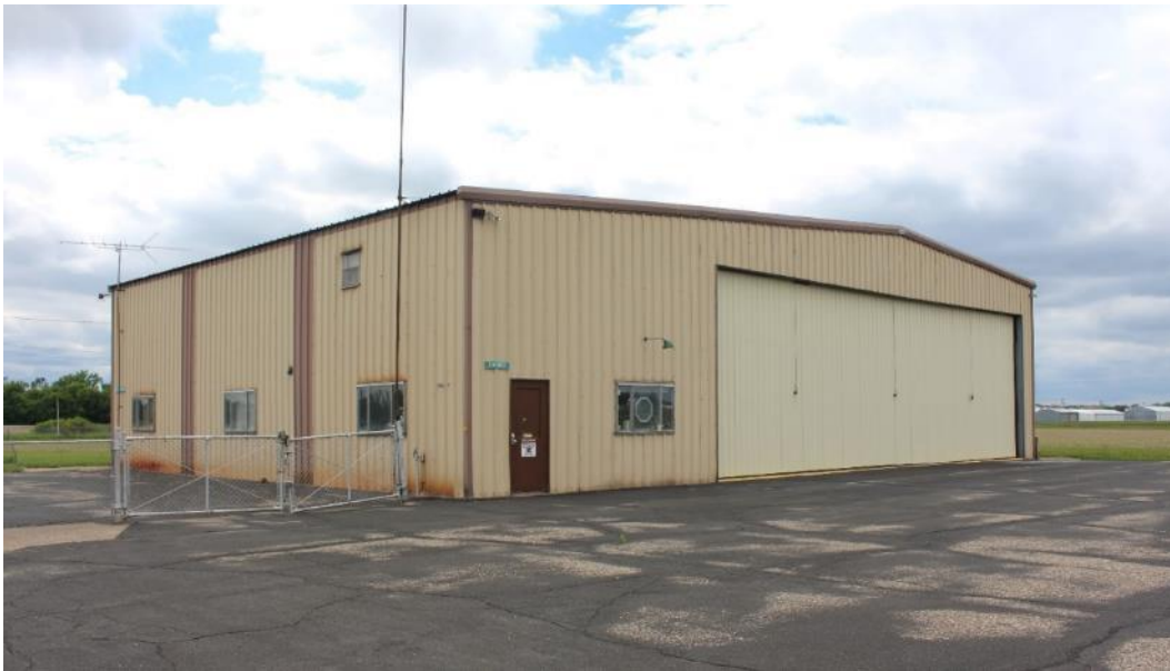
c.1970 south maintenance building, view facing southwest.
