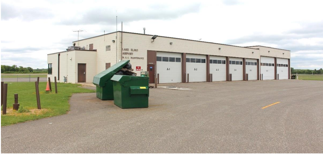
c. 1980 Lake Elmo MAC maintenance building, view facing southeast.
