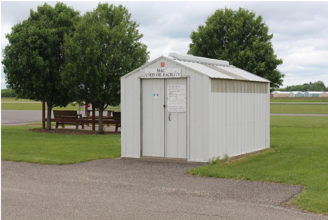
Used Oil Facility adjacent to MAC Maintenance Building.
