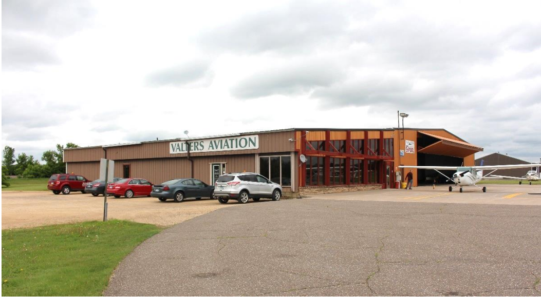
Valters Aviation Building, view facing northeast.
