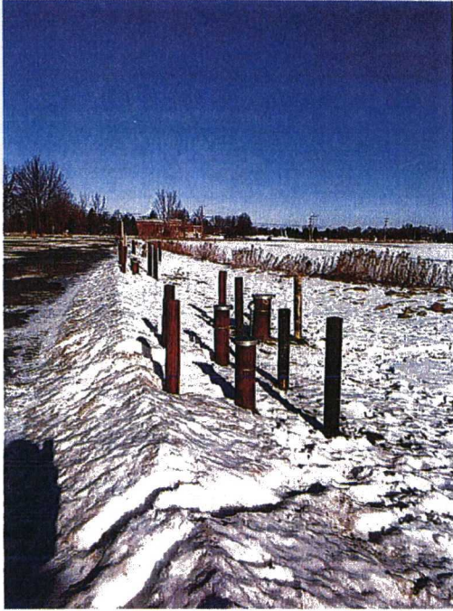
Monitoring wells along east edge of source area; view north
