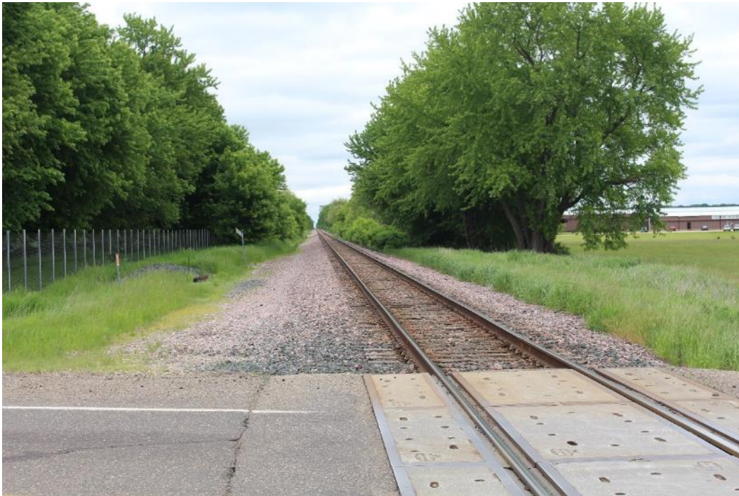
Union Pacific Railroad at intersection with Manning Avenue N.
