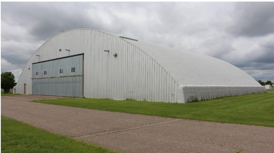
Large c.1970 Quonset Hangar, view facing north.
