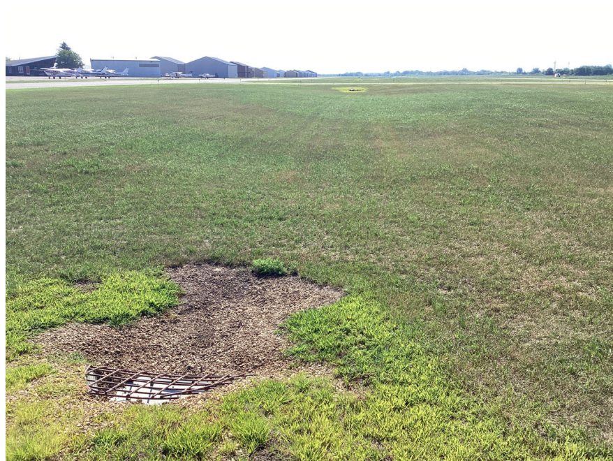
Photo 68. General site at culvert. View to the northeast.
