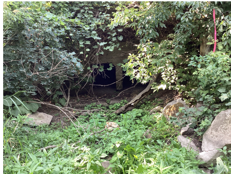
Photo 58. Double box culvert under railroad. View to the west.
