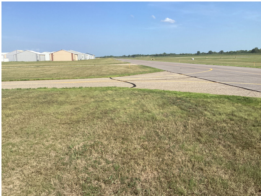
Photo 29. General site, north hangar area. View to the southeast.
