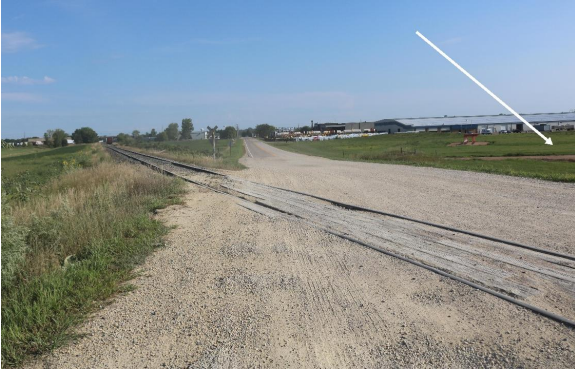
Figure 3. The MStPR&DETC Railroad Corridor at its crossing with Highview Avenue within the APE. The end of the runway is identified by the white arrow. View facing north.
