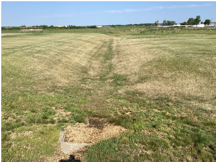
Photo 65. General site at swale. View to the southwest.
