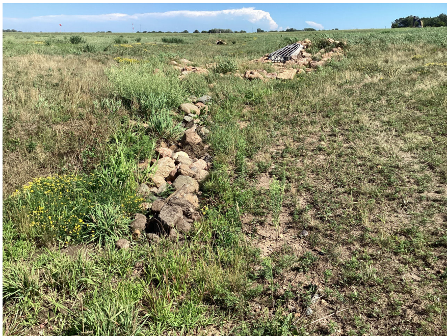
Photo 35. Culvert exit and rip rap drain. View to the southeast.
