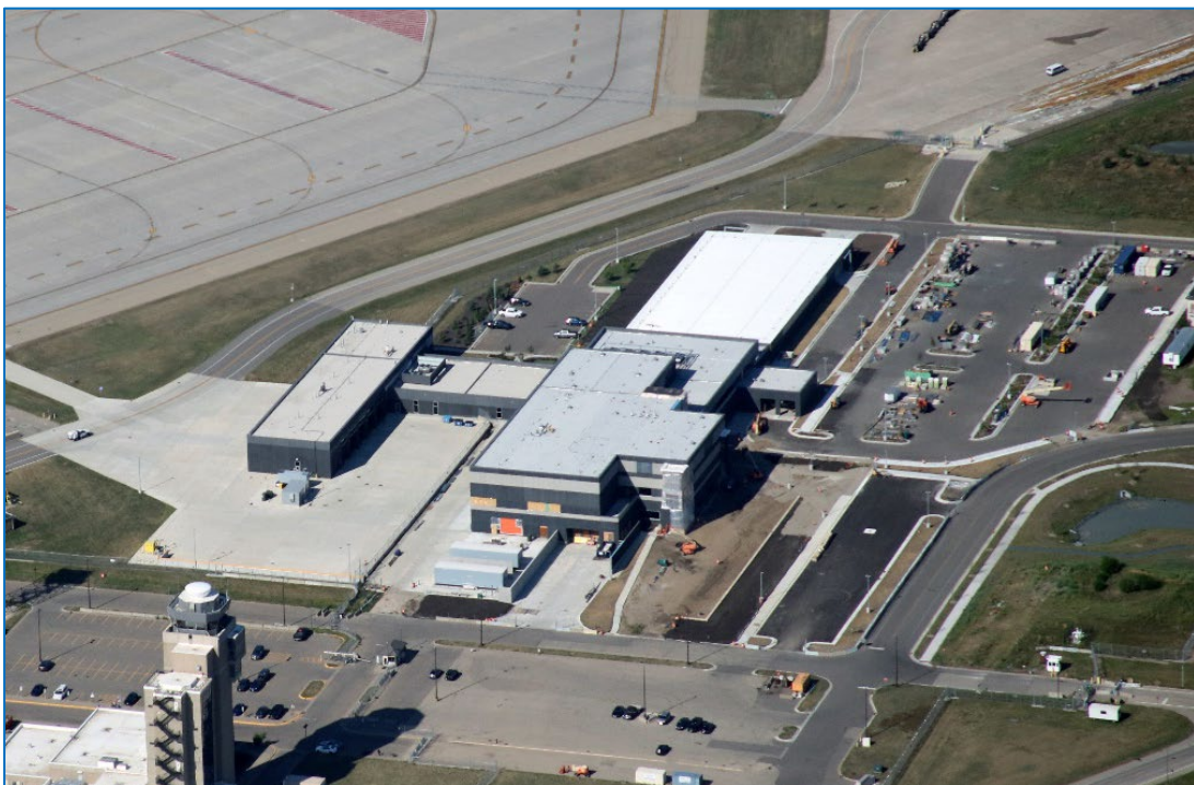
MSP Public Safety and Operations Center Construction
